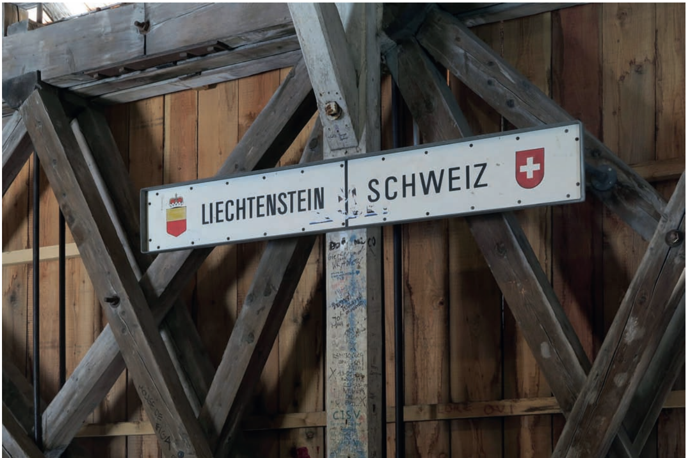
Rheinbrücke Sevelen-Vaduz. Bildnachweis: By Kecko from Northeast corner of, Switzerland (Wikimedia Commons).
